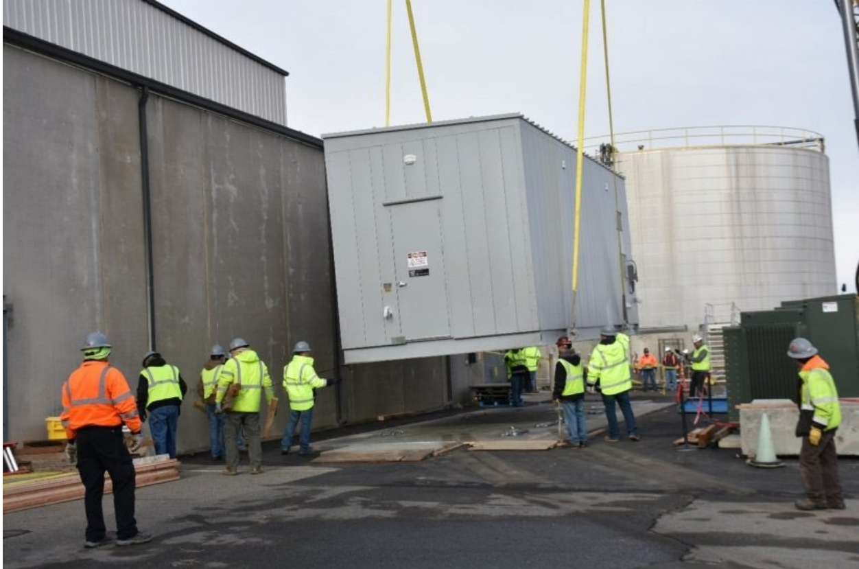
Equipment in this portable electrical facility will distribute additional power needed to run the many upgrades at the Effluent Treatment Facility.
