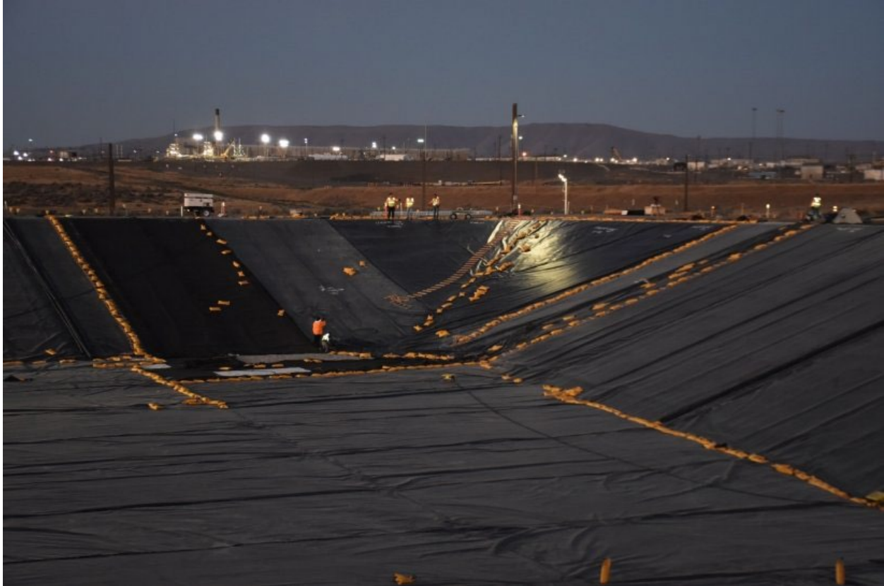
Crews with Washington River Protection Solutions work on the second of two liner systems at Liquid Effluent Retention Facility Basin 41 on the Hanford Site.
