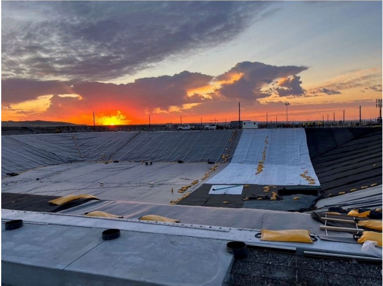
Liquid Effluent Retention Facility Basin 41 on the Hanford Site is one of four basins, each capable of holding nearly 8 million gallons of wastewater.
