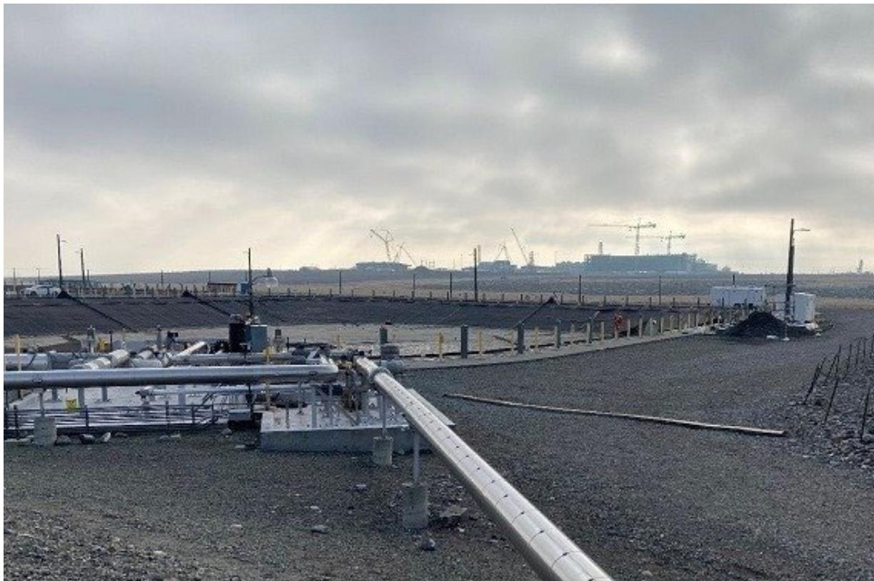
**During Hanford's Direct-Feed Low-Activity Waste Program treatment operations, the Waste Treatment and Immobilization Plant, background, will feed liquid waste to the Liquid Effluent Retention Facility, foreground, through a primary transfer line pictured.**
