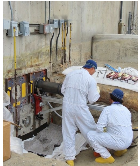
Washington River Protection Solutions workers install three new wall nozzles connecting new transfer lines to the 242-A Evaporator pump room on the Hanford Site.
