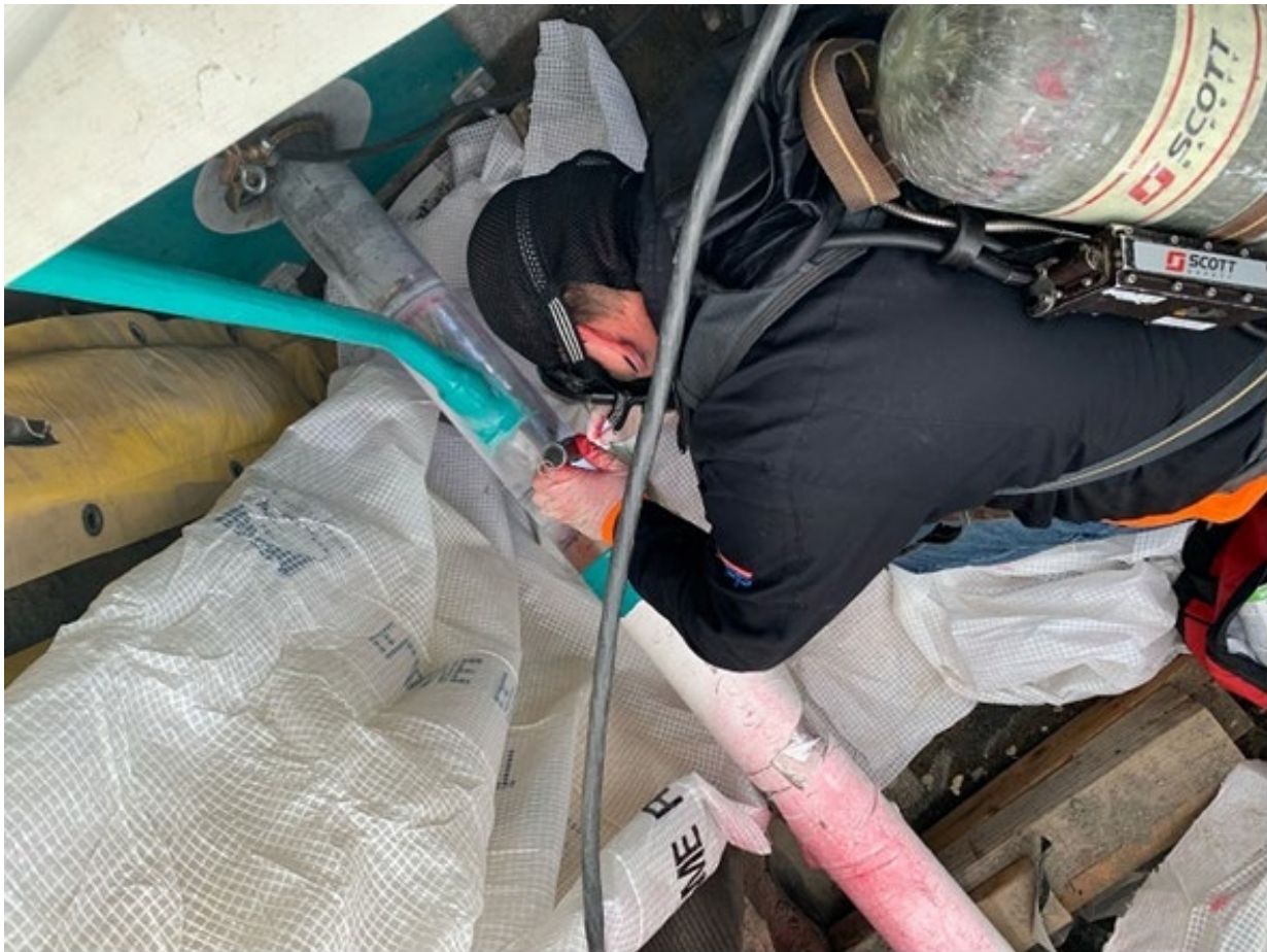
A worker installing new waste transfer lines between large, underground tanks and Hanford's evaporator facility welds a secondary encasement on one of the lines.
