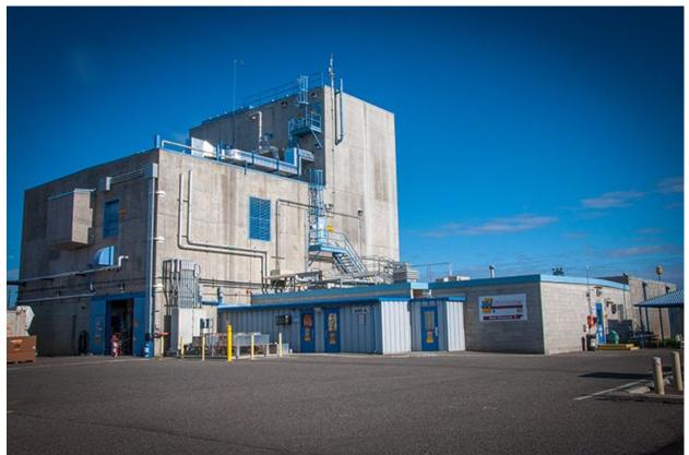
The 242-A Evaporator removes water from tank waste and reduces the volume stored in the double-shell tanks to make room for waste retrieved from single-shell tanks until it can be permanently disposed.
