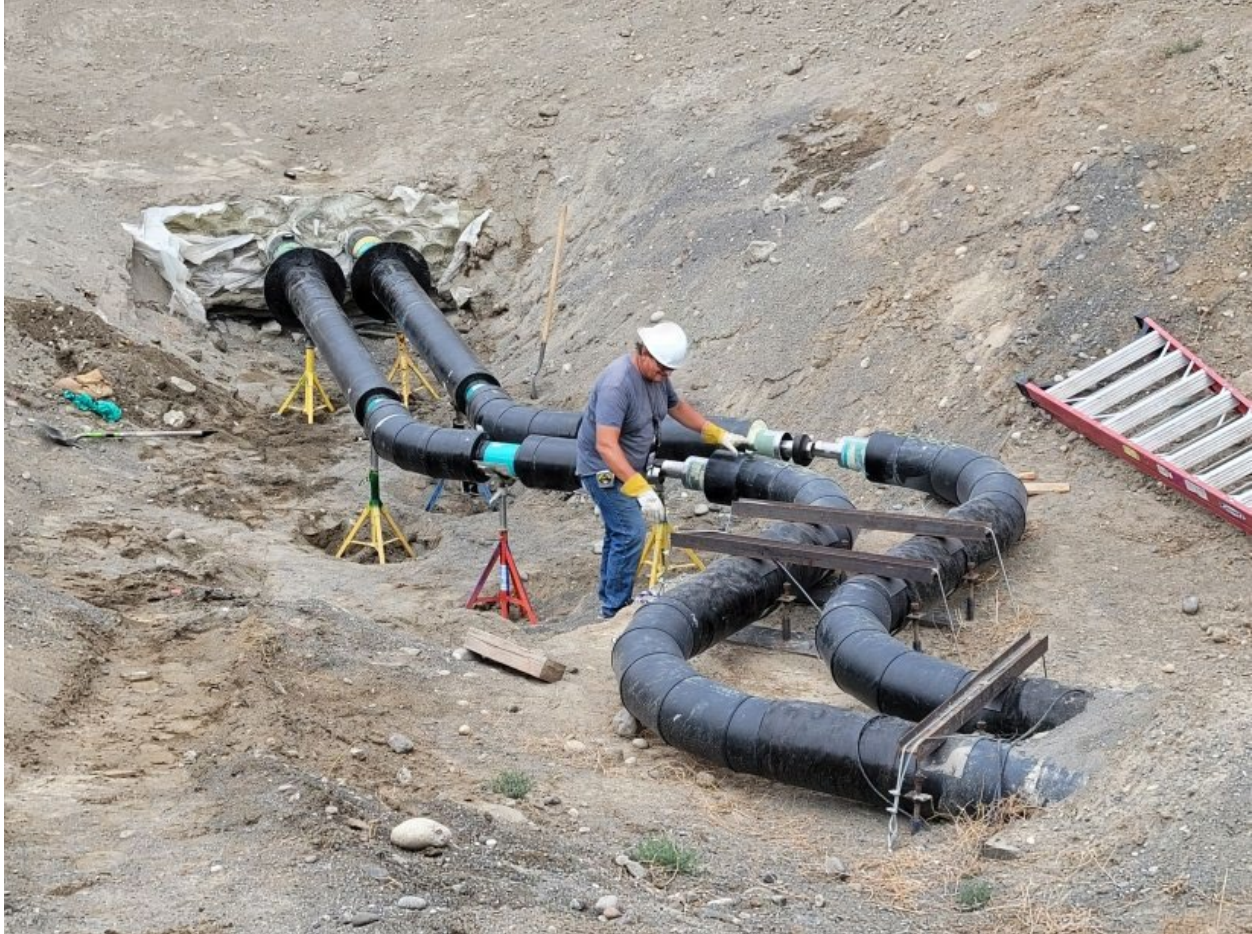
In August 2021, workers made the final welds on the transfer line connecting the Hanford Site's tank farms to the Waste Treatment and Immobilization Plant.
