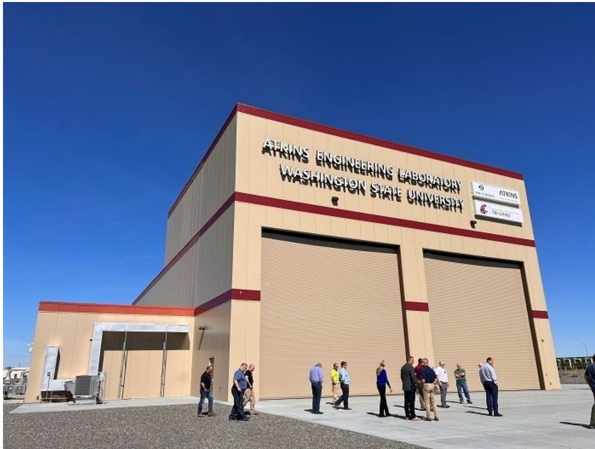
Representatives from the Office of River Protection and broader DOE tour the Low-Activity Waste Melter Assembly, Storage and Transportation facility near the Hanford Site prior to the installation of steel rails outside of the bay doors.
