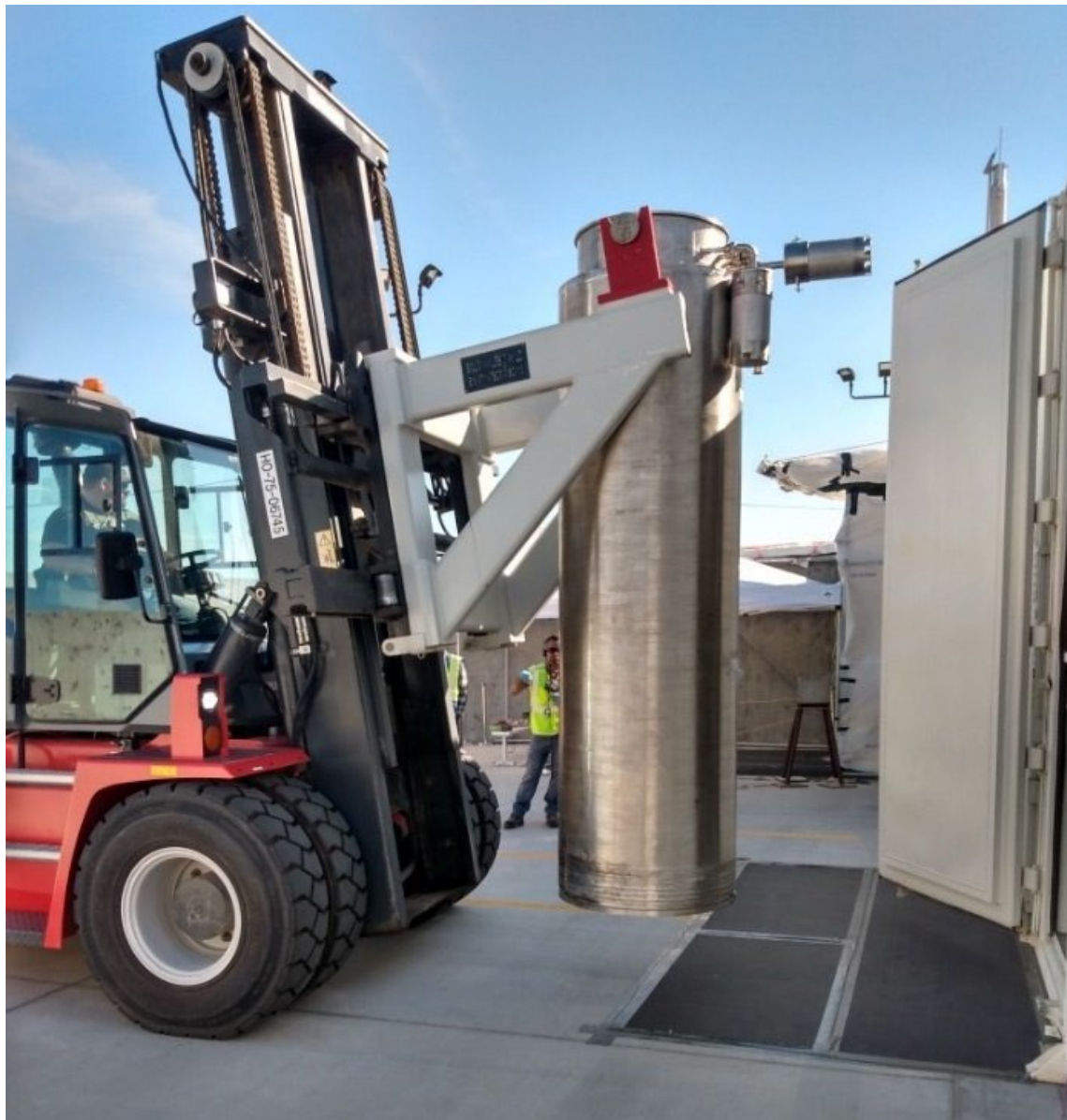
Workers with Hanford Site tank waste contractor Washington River Protection Solutions remove the first cesium-filled ion exchange column from the Tank-Side Cesium Removal System.
