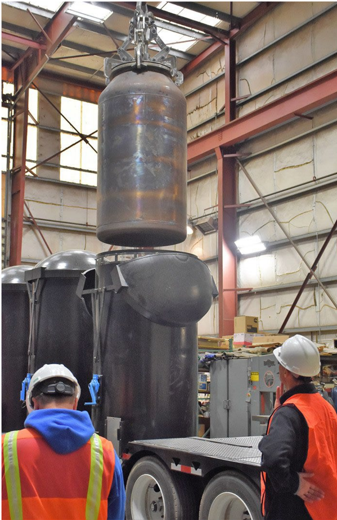
The immobilized low-activity waste transporter system consists of a trailer with three pallets, which will be loaded with containers of tank waste mixed with hot glass for transport to Hanford's Integrated Disposal Facility.
