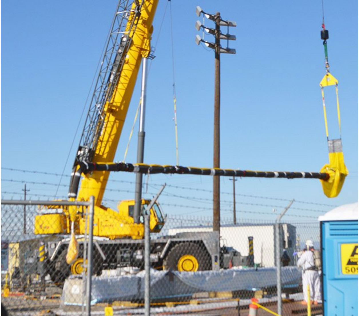
With help from a second crane, the outdated pump is lowered horizontally toward the disposal box.
