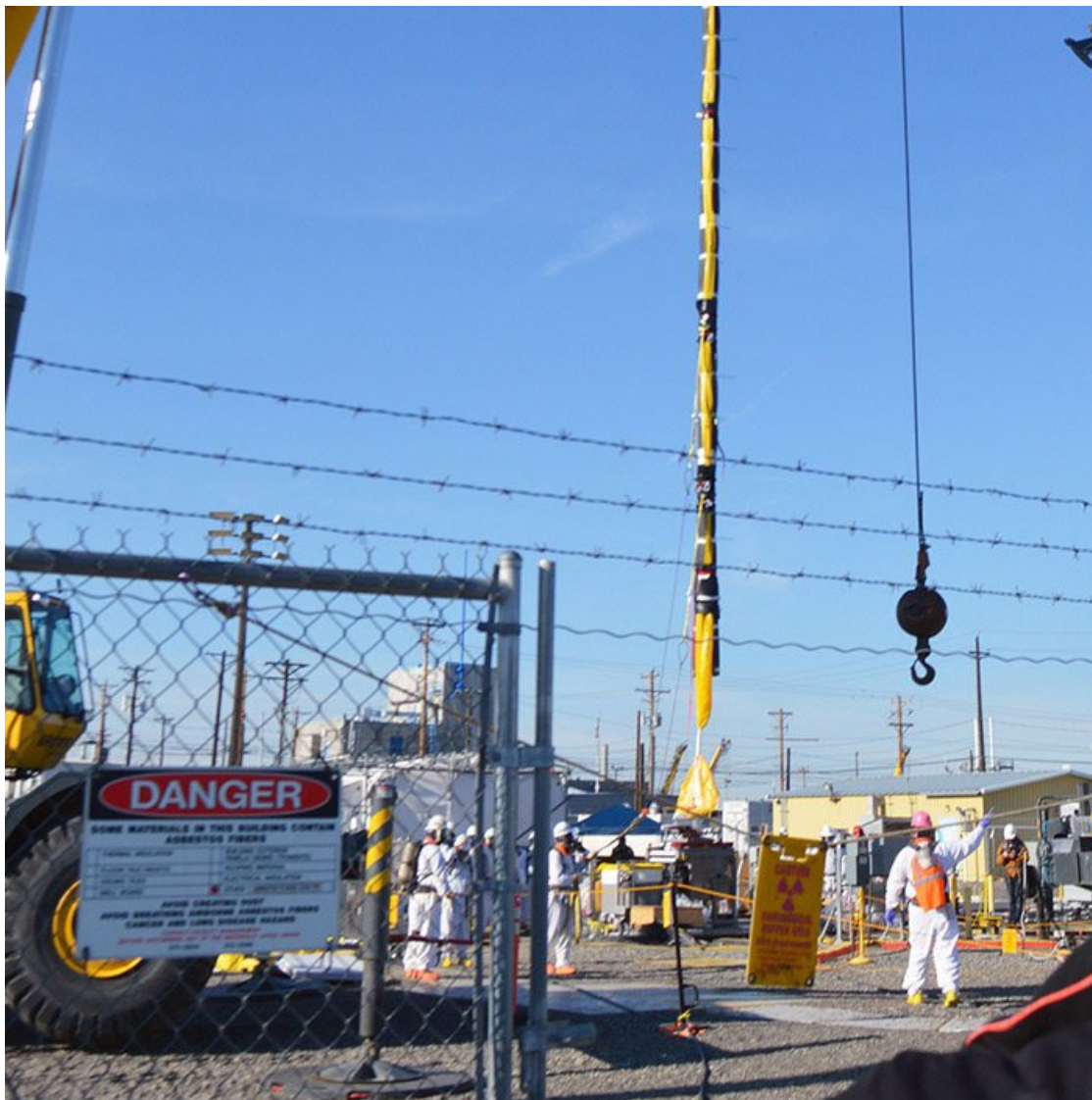
The crane that pulled the pump at the AP Farm eases it toward the disposal box.
