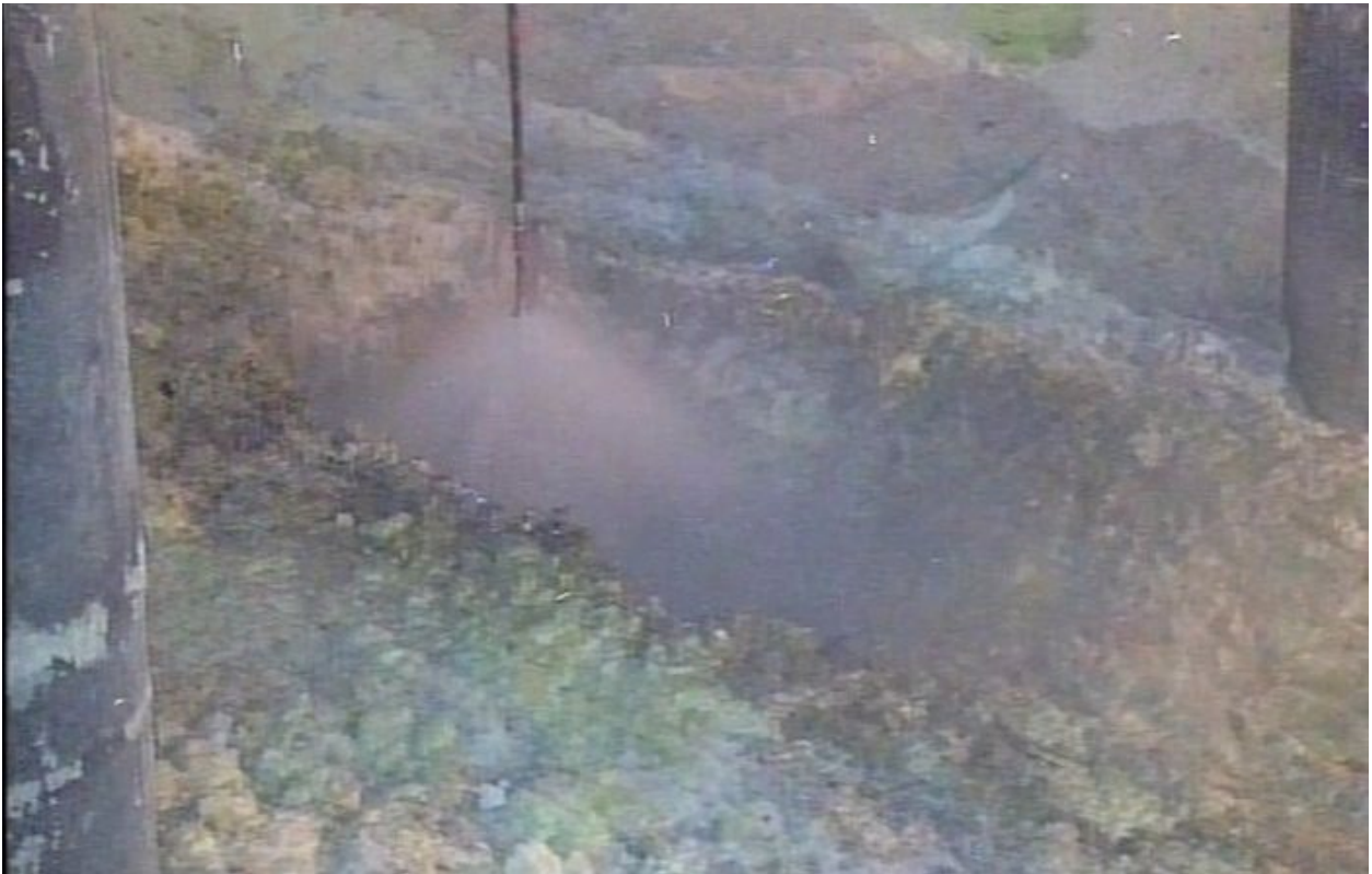
A tool known as a "wolverine" used water pumped through high-velocity nozzles to create a hole in the saltcake of Tank AX-101 to allow a sluicer to be installed.
