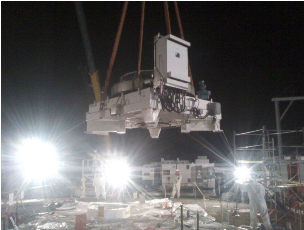
MARS-V being installed into Tank C-105.
