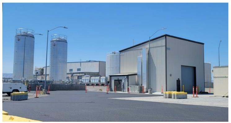
The Hanford Site's Effluent Treatment Facility has been expanded to handle almost 7 million more gallons of wastewater per year when Hanford's Waste Treatment and Immobilization Plant begins treating waste from large underground tanks.
