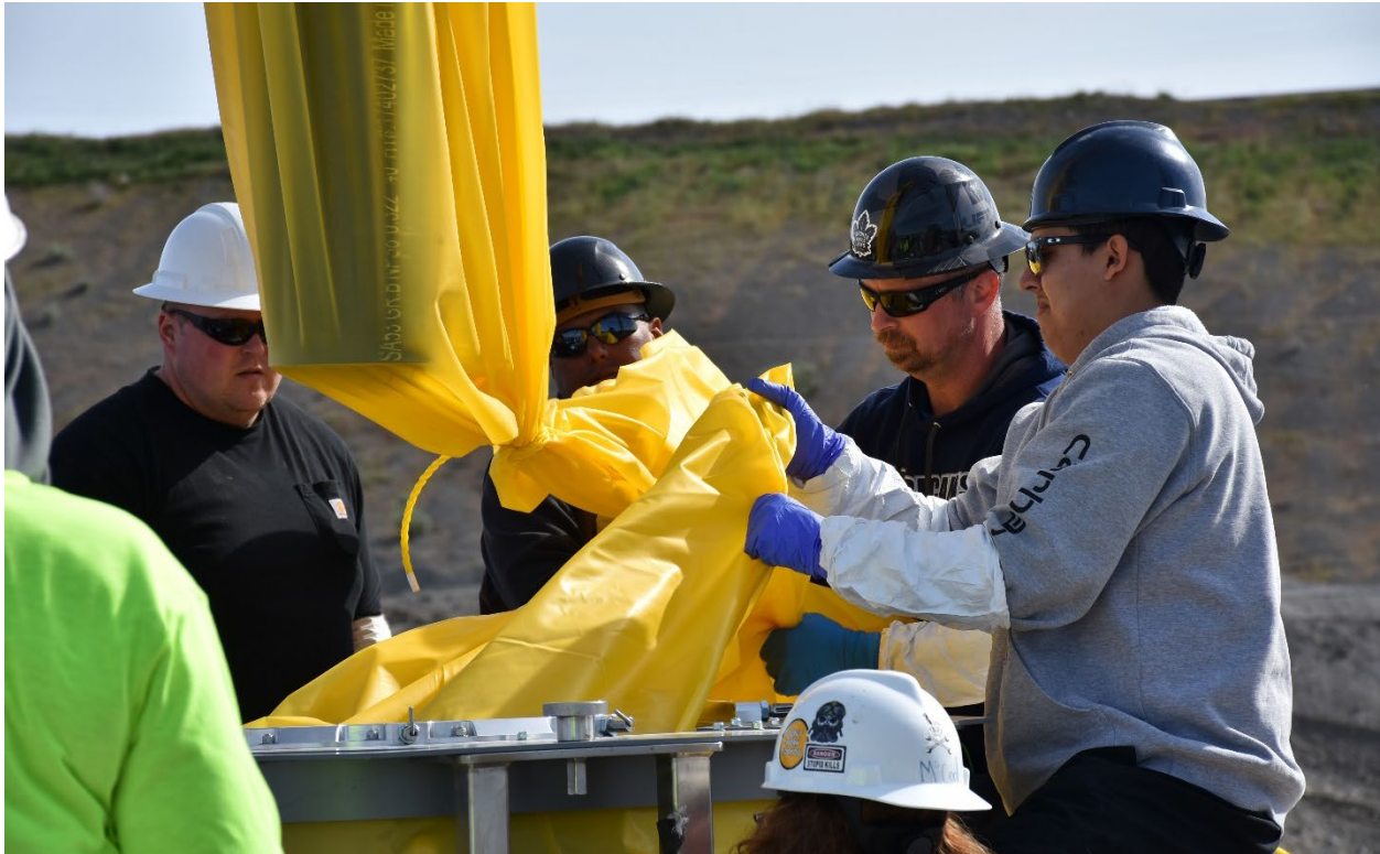
Crews with U.S. Department of Energy Office of Environmental Management contractor Washington River Protection Solutions demonstrate bagging and retrieving a hydraulic pump from a tank in a simulated, nonradioactive environment, then packaging it for disposal after its pipes are drained of fluid.
