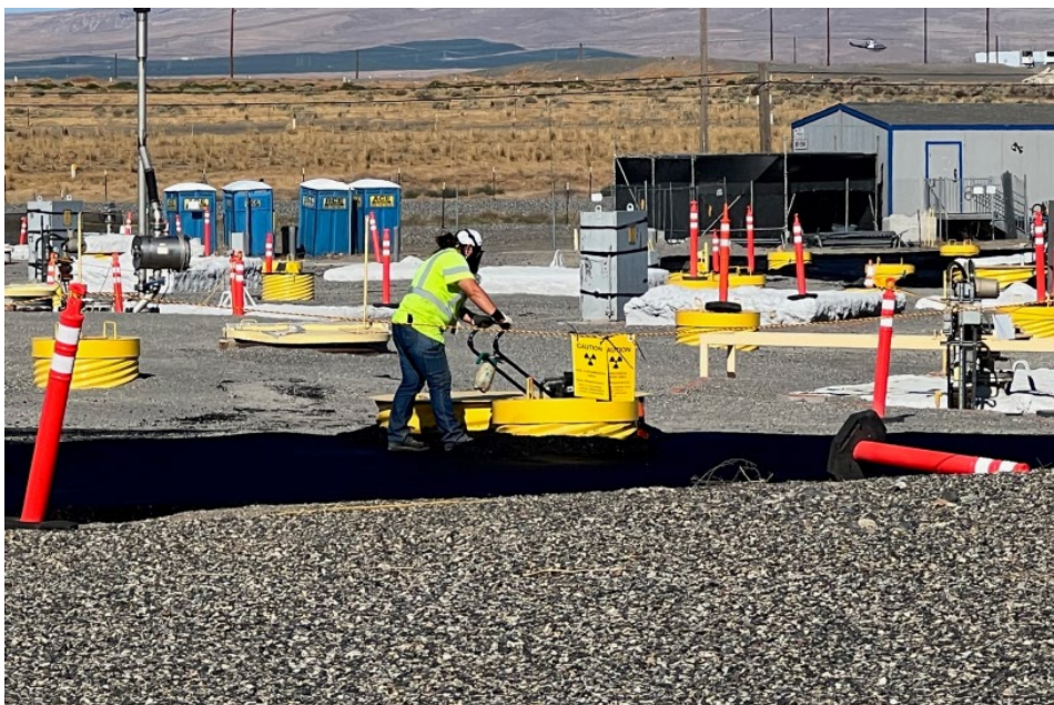
Crews operate compactors to level and compress surface barrier asphalt in tight areas around infrastructure at the U Tank Farm on the Hanford Site.
