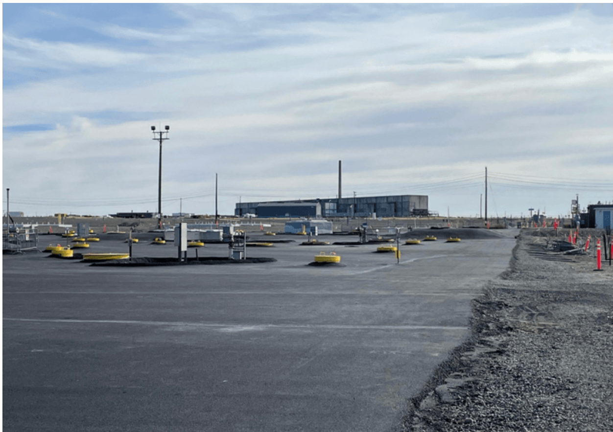
A new interim surface barrier recently installed over the Hanford Site's U Tank Farm.
