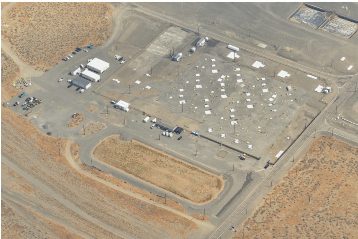
An aerial of the Hanford Site's U Tank Farm and its runoff basin before workers installed the surface barrier.
