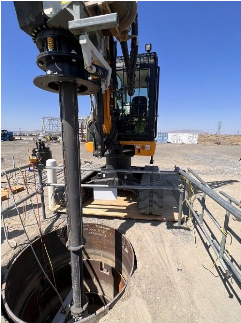
Workers use the Tank Dome Core Cutting System, a modified drilling machine that will create an access hole in the top of an underground waste-storage tank where workers will install equipment to retrieve radioactive and chemical waste from the tank.
