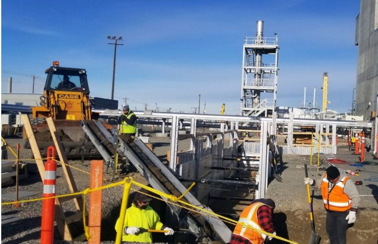
A shoring system and innovative conveyor belt system used to move soil out of trenches helped protect workers manually digging the trenches to replace waste transfer lines on the Hanford Site earlier this year.
