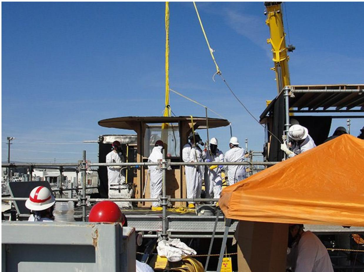
A Hanford Site team created unique tools to remove a radiologically contaminated thermocouple from single-shell tank AX-103. The team built a radiation-shielding box and remote extension tools to allow workers to complete the task more safely.
