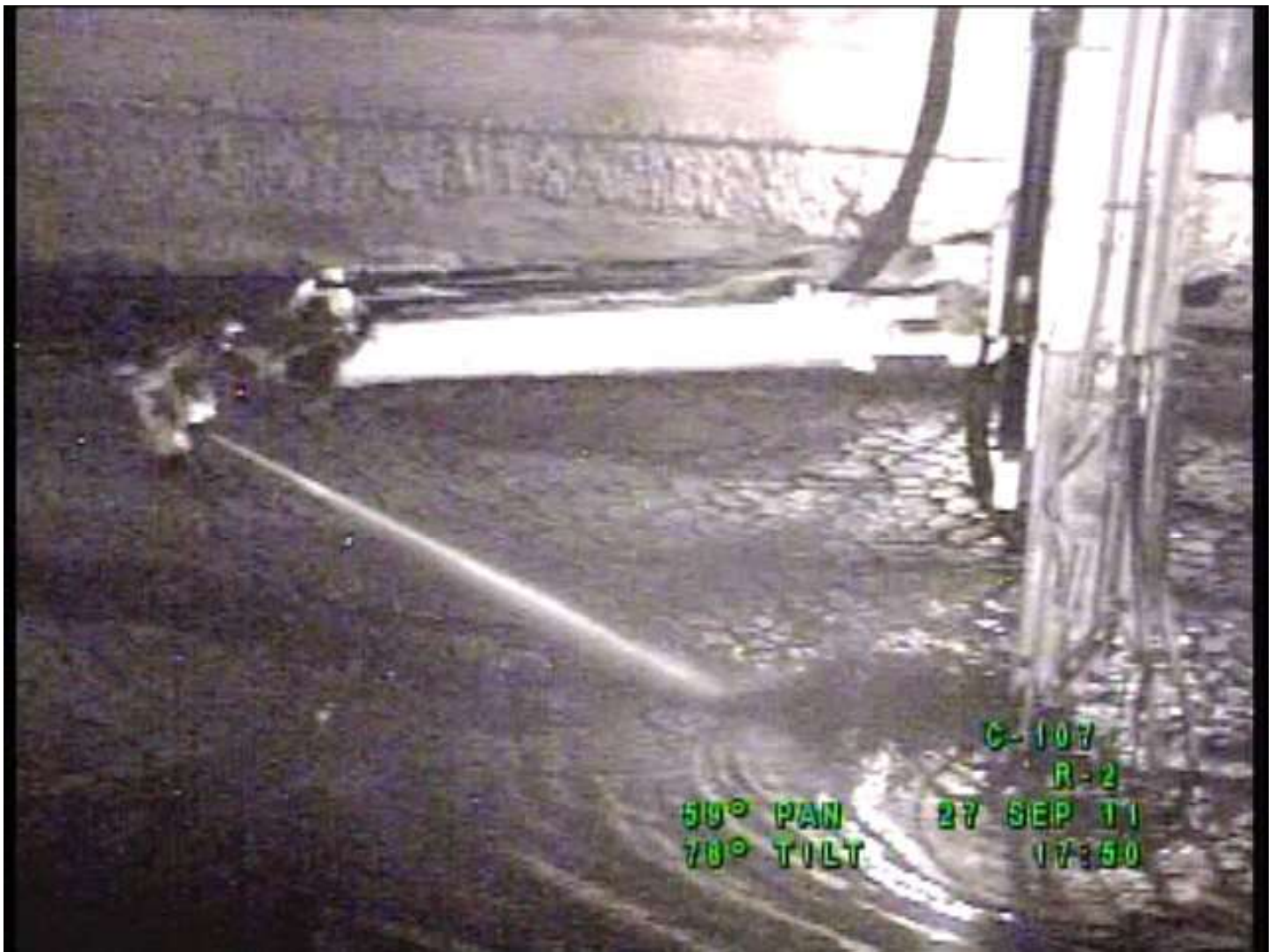
The Mobile Arm Retrieval System, the largest robotic arm ever inserted into a Department of Energy waste storage tank, is at work at Hanford removing 253,000 gallons of waste from single-shell Tank C-107.
